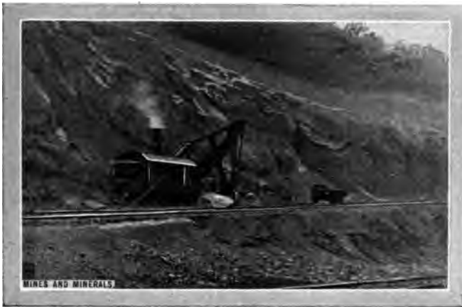
FIG. 3—Steam Shovel Loading Iron Ore.
